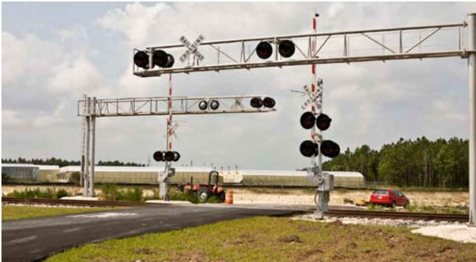
Railroad Crossing at 441
