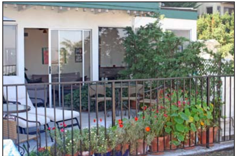
Private rooftop deck
